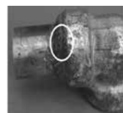
SS Wash water line
