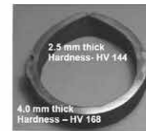
Cross section boiler tube
